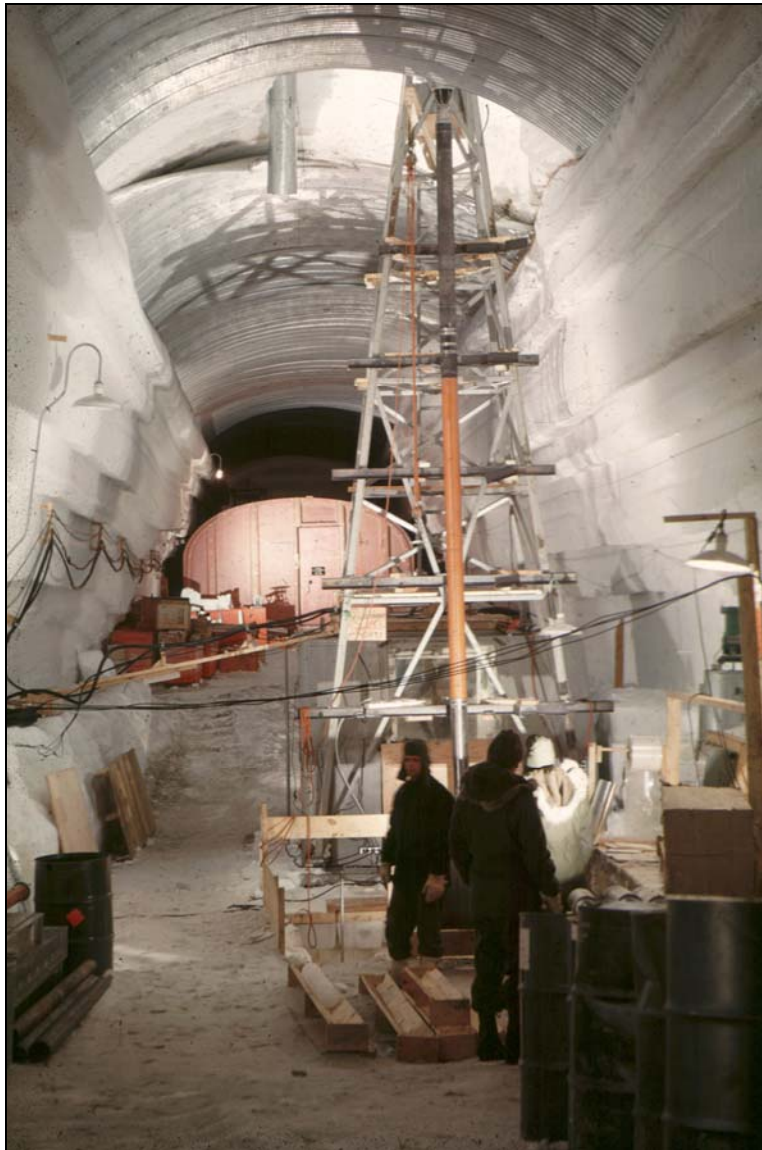
Figure 17. Thermal coring rig in Trench 12 at Camp Century, 1964. Senior Engineer H. Ueda (back to camera) and Specialist W. Vest are standing next to the ice core increments in carriers. The orange composite building at the rear is the driller's work shop.
