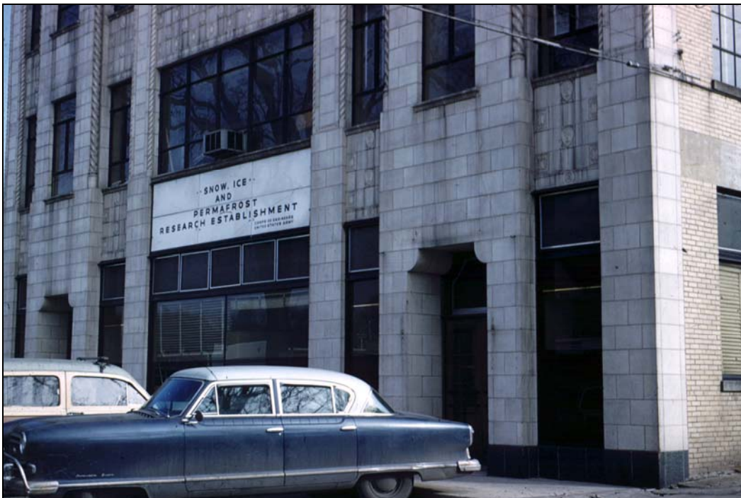
Figure 1. SIPRE Administration and Laboratory Building, Wilmette, IL, 1956.
