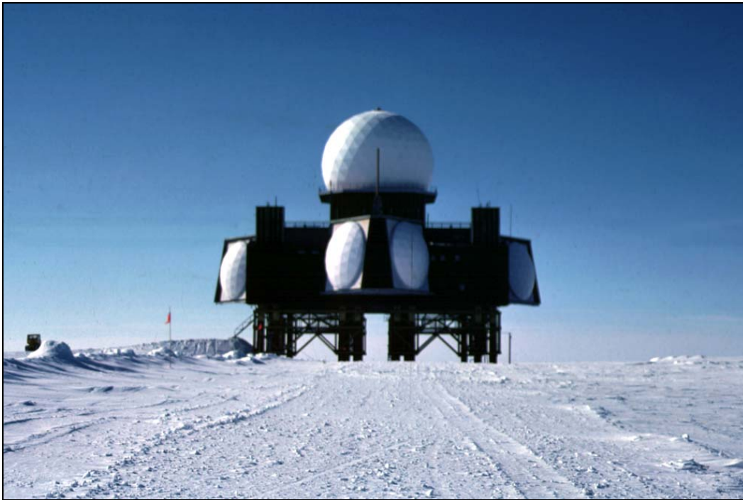
Figure 25. Dye 3, Greenland radar and communications site, 1980. The top of the structure is approximately ten stories high; at the left side is a sloping staircase, about 2 1/2 stories high, for pedestrian access to the building.
