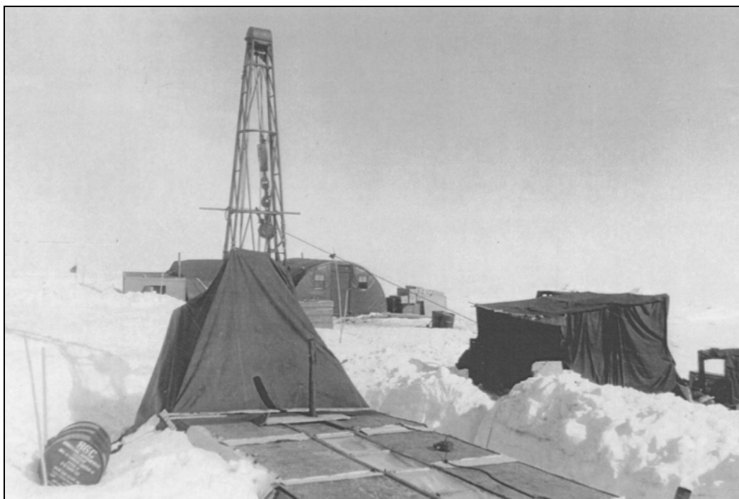
Figure 7. Surface view of the Site 2 drill tower and support structures, 1957. The Jamesway shelter in the background served as a heated office and warm laboratory at the drill site.
