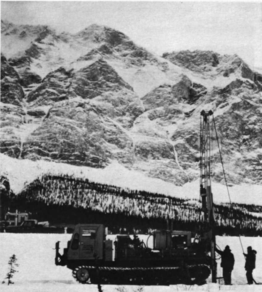
Augering holes for installation of thermocouples, trans-Alaska pipeline haul road.
