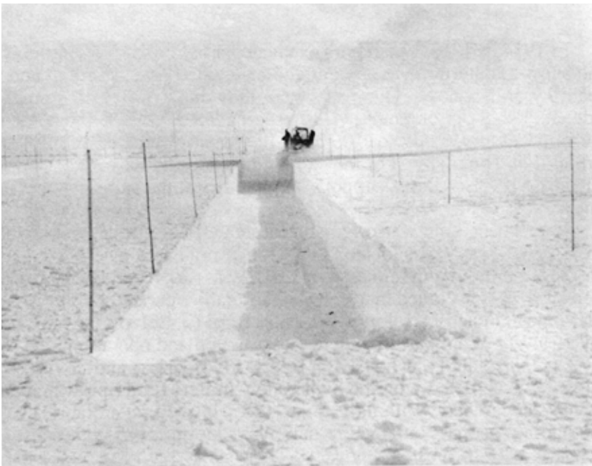
Peter Plow starts to cut ramp for Project 33 at Camp Century, Greenland.
