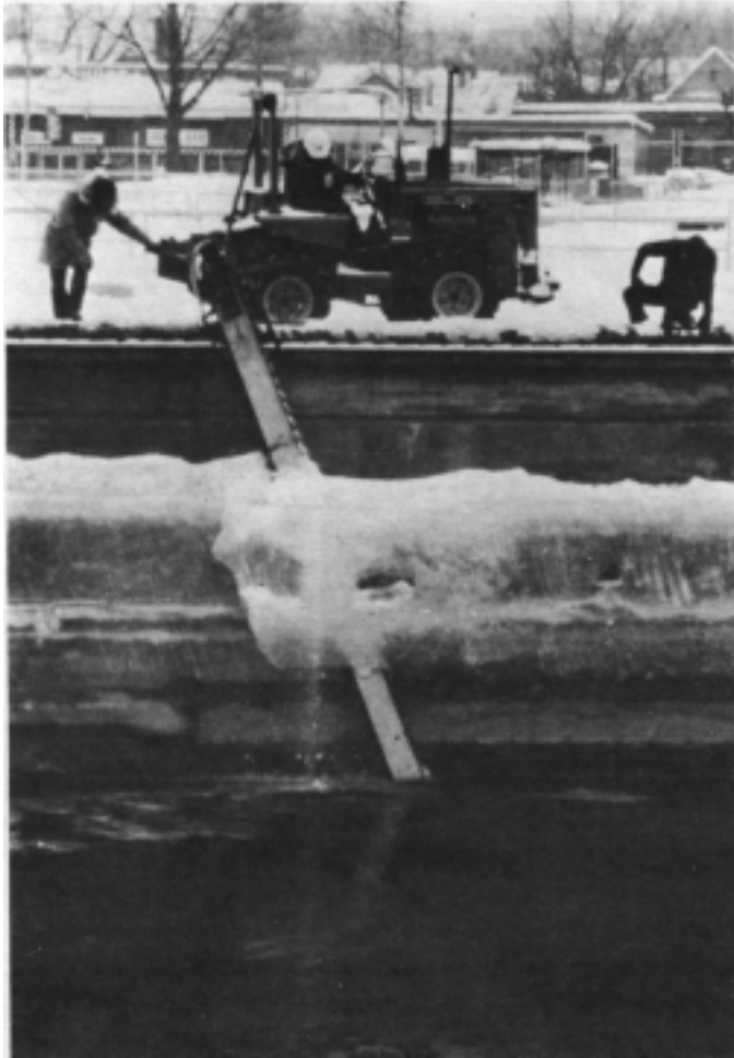
Large saw used to cut ice from lock walls at Sault Ste. Marie, Michigan.
