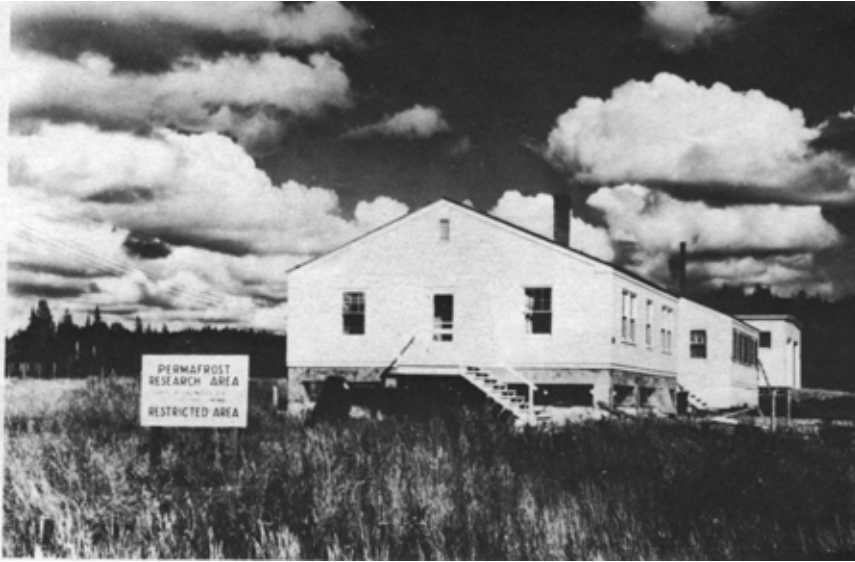
Experimental foundations at Alaska Field Station.
