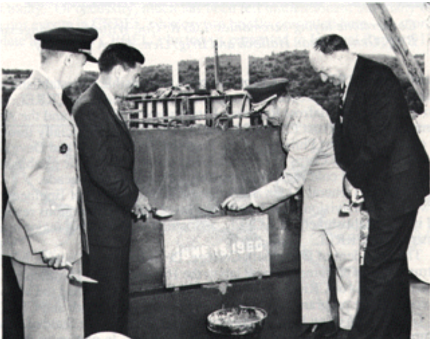
Cornerstone laying ceremonies. L to R: Brig. Gen. Duncan Hallock, Chief, Research and Development Division, Office of the Chief of Engineers, Washington, D.C.; Gov. Wesley Powell, State of New Hampshire; Brig. Gen. Alden K. Sibley, Division Engineer, New England Division, U.S. Army Corps of Engineers; and Dr. John Sloan Dickey, President, Dartmouth College.
