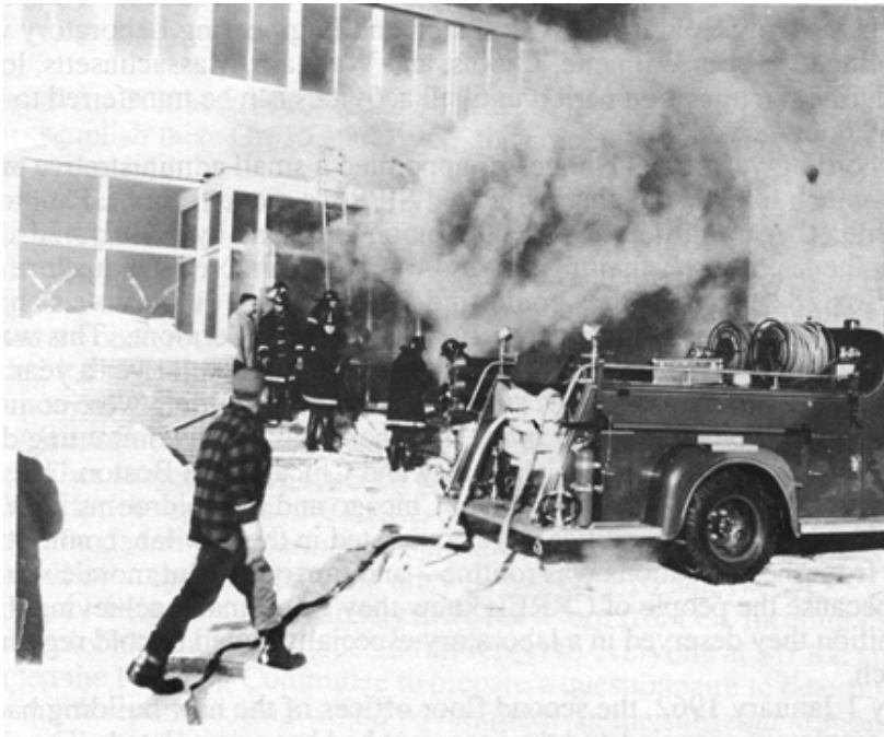
Smoke at CRREL's front entrance during construction fire, 4 January 1962.
