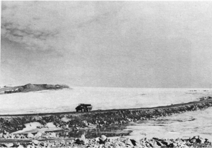
Height of fill on ramp road, August 1955.
