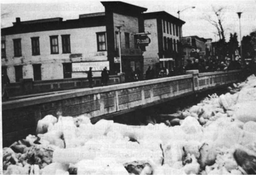
Bridge endangered by ice jam (Lancaster, New Hampshire).
